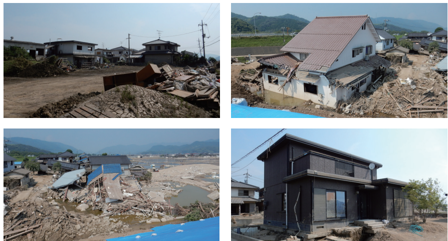
Figure 1: RMS Field Reconnaissance following Non-Typhoon Flooding in July 2018
