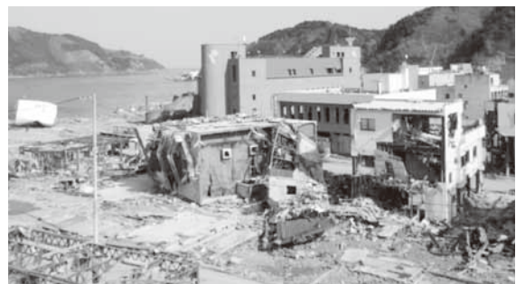
Figure 2. Devastation in Onagawa, showing heavy, mid-rise concrete structures toppled due to the tsunami waves following the 2011 Great East Japan Earthquake (Source: RMS)
